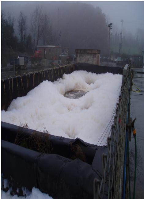
percolates through the landfill it dissolves soluble organic material so that it is highly polluting when it emerges from the landfill. Therefore the leachate must be treated before it can be discharged.
