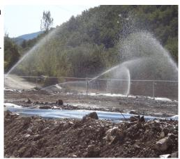
been specially selected for their ability to efficiently break down the many different compounds contained in oil products. The use of BFL 6000HC together with nutrients will accelerate the degradation of hydrocarbons so that the toxicity of the soil is eliminated. BFL 6000HC uses only harmless, natural micro-organisms that deal with the contamination by degrading the hydrocarbons to  $CO_2$  and  $H_2O$  in an environmentally acceptable way.
